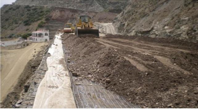
Levelling/compaction of the filling, gabions being used as well as temporary formwork, Enka-Tex pending layer on the gabions
