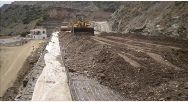
Levelling/compaction of the filling, gabions being used as well as temporary formwork, geotextile pending layer on the gabions
