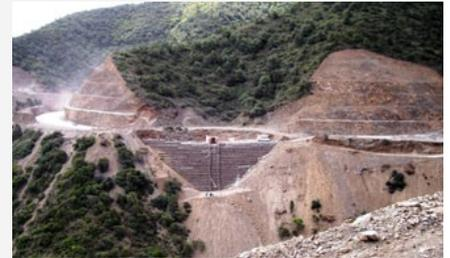
EnkaGrid retaining solution minimised the load on top of the existing slopes
