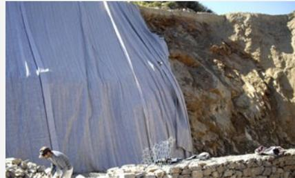
EnkaDrain in very aggressive conditions of use (tensile strength and puncture resistance)
