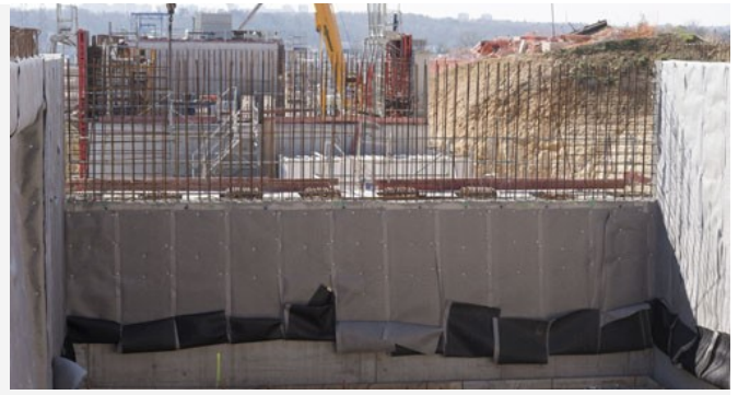
No loss due to overlapping: EnkaDrain is provided with 10 cm overlap of fleeces
