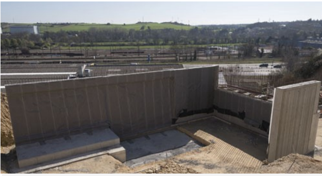
Overview of the abutment
