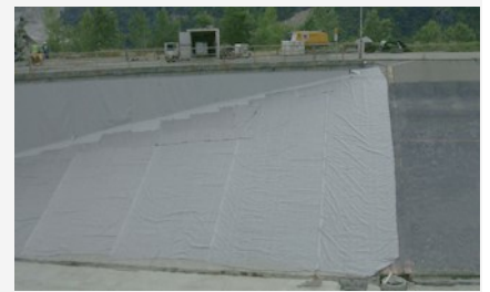
EnkaDrain Wide on a side slope
