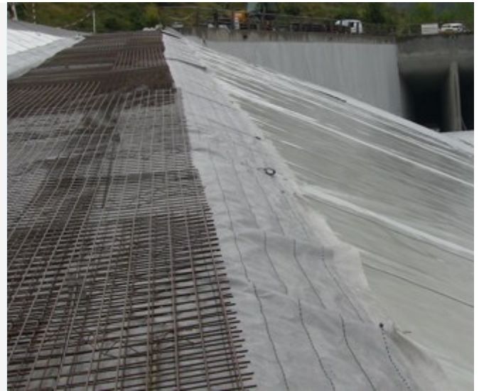
EnkaDrain Wide providing protection on the access ramp.
