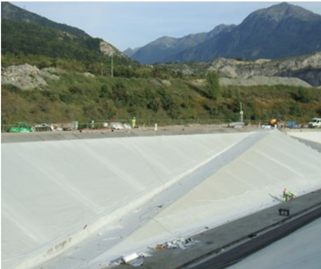
Access ramp close to the upstream inlet.
